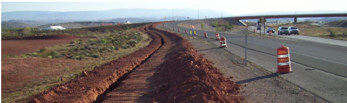
Exhibit 7 – Trench for Fiber Optical Cable along I-15
